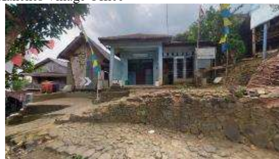
Figure 12. Kanekes Village Office
