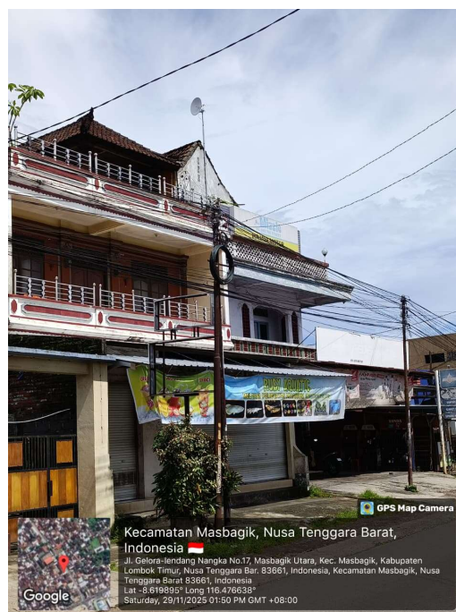
Figure 7. Signal Transmitting Antenna (Main1)
