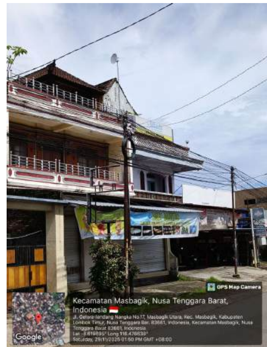
Figure 7. Signal Transmitting Antenna (Main1)
